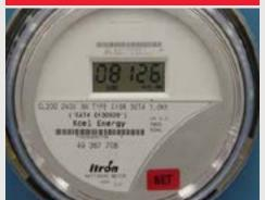
This net meter rolls backwards when your PV system is generating more electricity than you are using in your home and it rolls forwards when you are pulling electricity into your home from the grid. During a 24 hour time frame this meter has the potential for back and forth motion. At the end of the billing cycle we use the meter reading to send you a net summary of your electric consumption or production.
